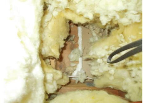
Air sealing top plates from the attic prior to blowing insulation has proven successful
