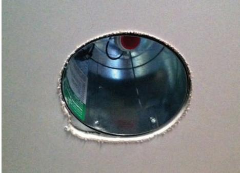
Ensure all recessed lights and exhaust fans are caulked at drywall when adjacent to unconditioned spaces.
