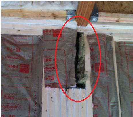
Check to ensure that steel beams connected to unconditioned space are air sealed prior to insulation. This is an ideal application for closed-cell foam.
